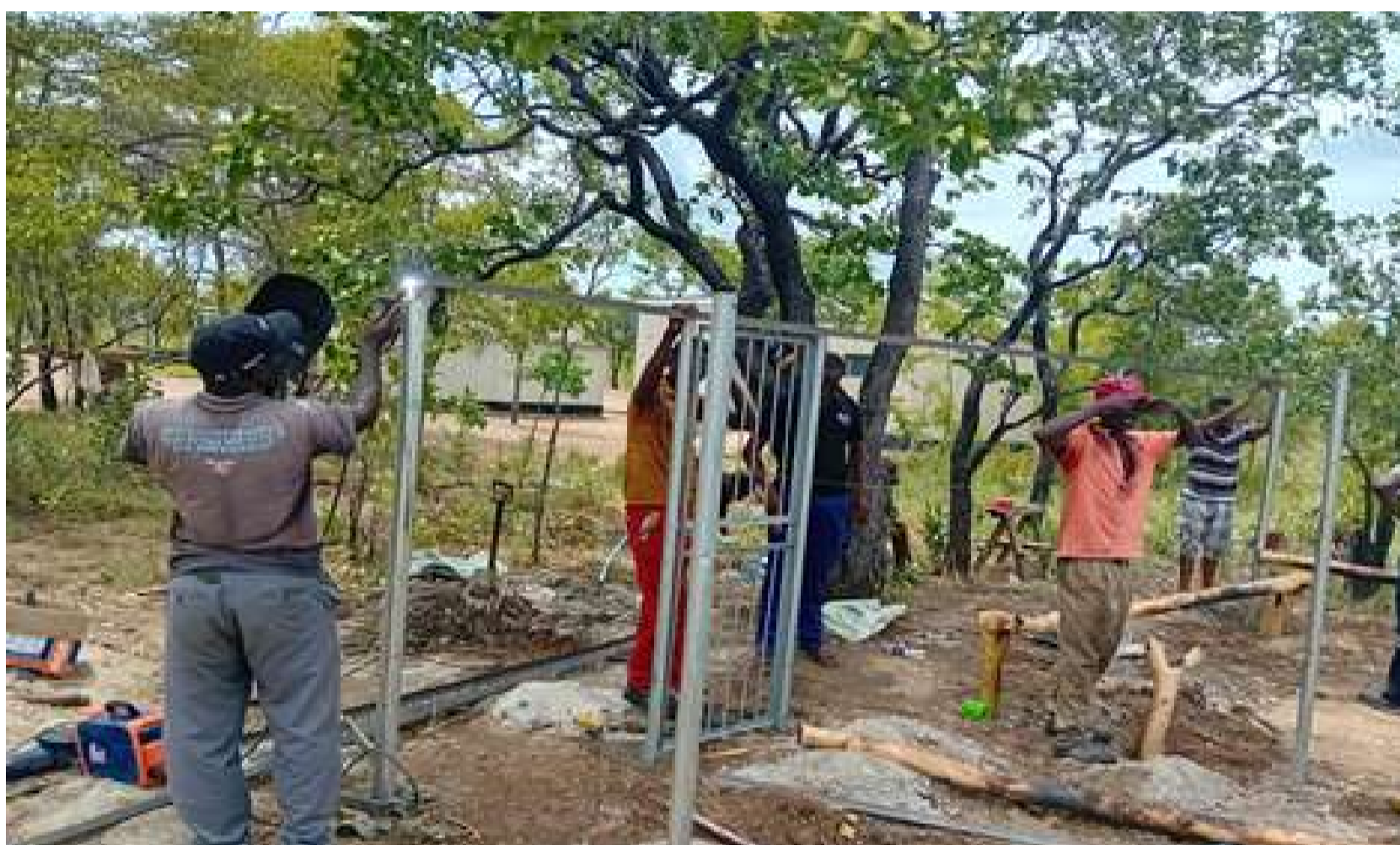
Contractor establishing Goat pen.
